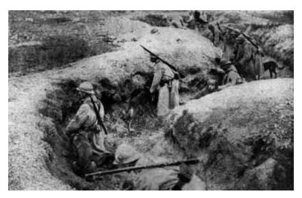
Trenches were not built in straight lines. This was so that if the enemy managed to get into the front line trench they would not have a straight firing line along the trench. Trenches were therefore built with alternating straight and angled lines. The traverse was the name given to the angled parts of the trench.
