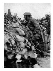
Sandbags were used to protect the soldiers from enemy rifle fire. They were, however, less effective in the event of shell fire. Sandbags were also sometimes placed in the bottom of the trench to soak up water.
